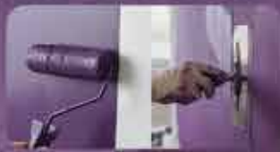
Apply Mobi Velvet Dream with roller and create effect by using trowel (2 to 3 coats)
