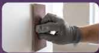
Prepare the wall by Sanding it with Sand Paper
